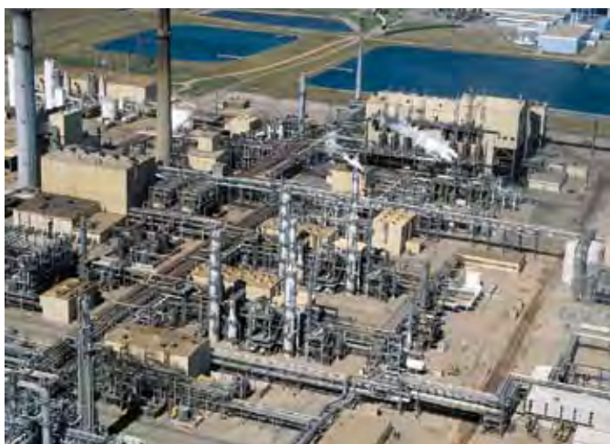
Figure 3.15 North Dakota coal gasification plant with 3.3 MtCO 2 yr -1 capture using a cold methanol, physical solvent process (cluster of 4 tall columns in the middle of the picture represent the H 2 S and CO 2 capture processes; part of the captured stream is used for EOR with CO 2 storage in Weyburn, Saskatchewan, Canada).
