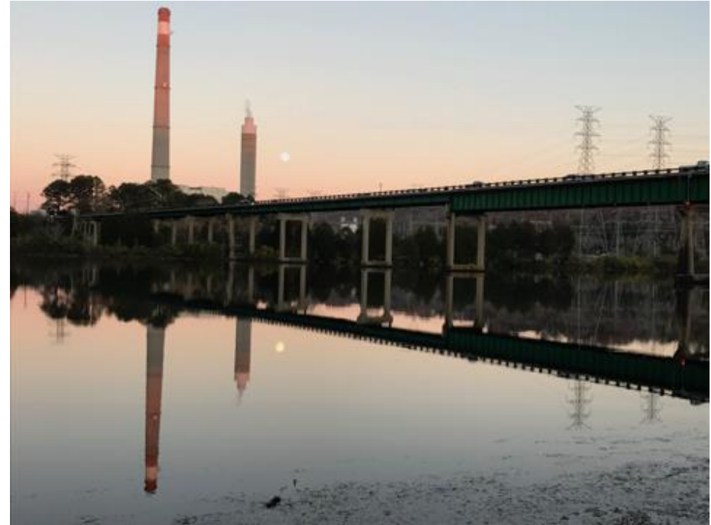
TVA Bull Run coal-fired power plant, with old & new stacks, retiring 2023. Oak Ridge, TN
