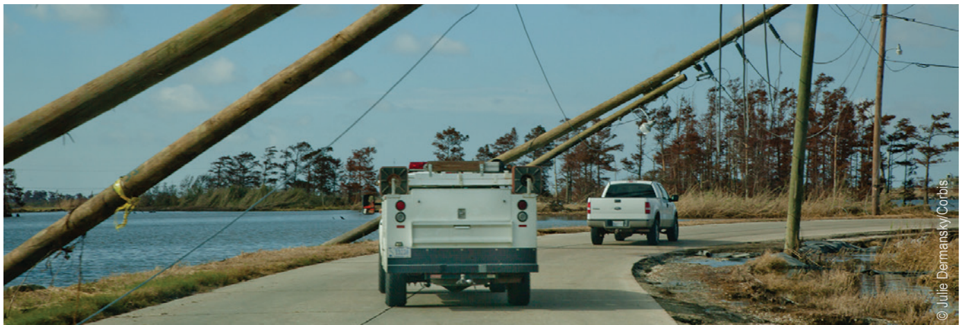
(Top) A truck gets stuck in the storm surge covering Highway 90 in Gulfport, Mississippi, during Hurricane Isaac. (Bottom) Power lines damaged in Plaquemines Parish, Louisiana, by Hurricane Isaac. September 3, 2012.
